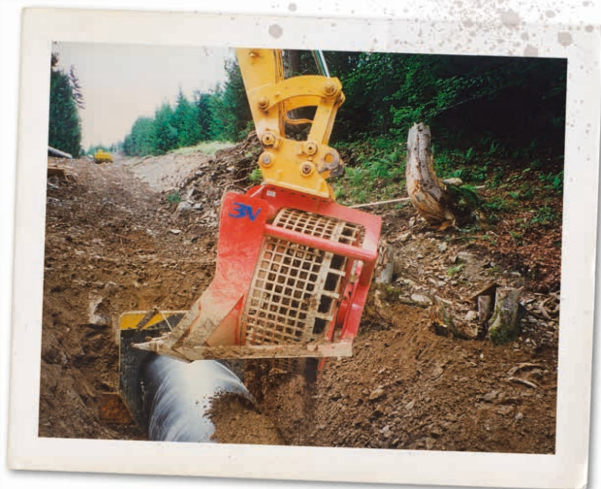
1994 Innsbruck, Austria Mountain pipeline coverage
